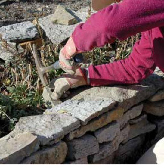
*For a stable wall, it may be necessary to fill gaps with fragments of stone.*
